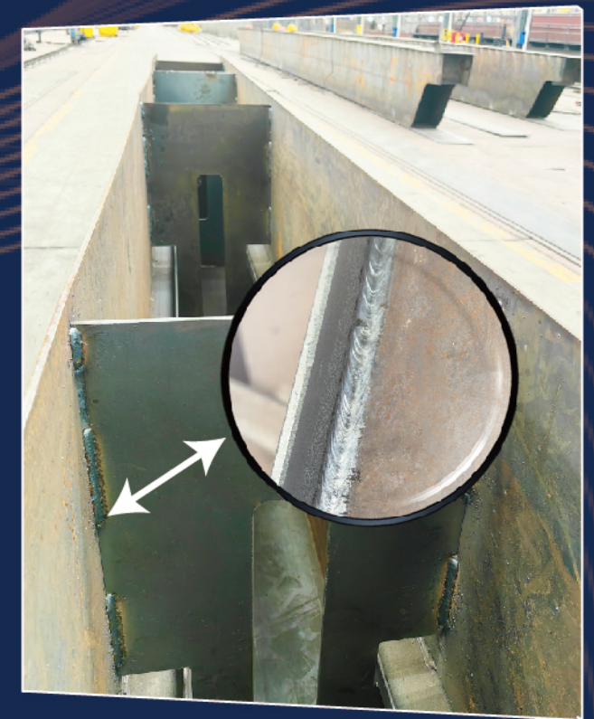
Main Girder Internal Welding Process
