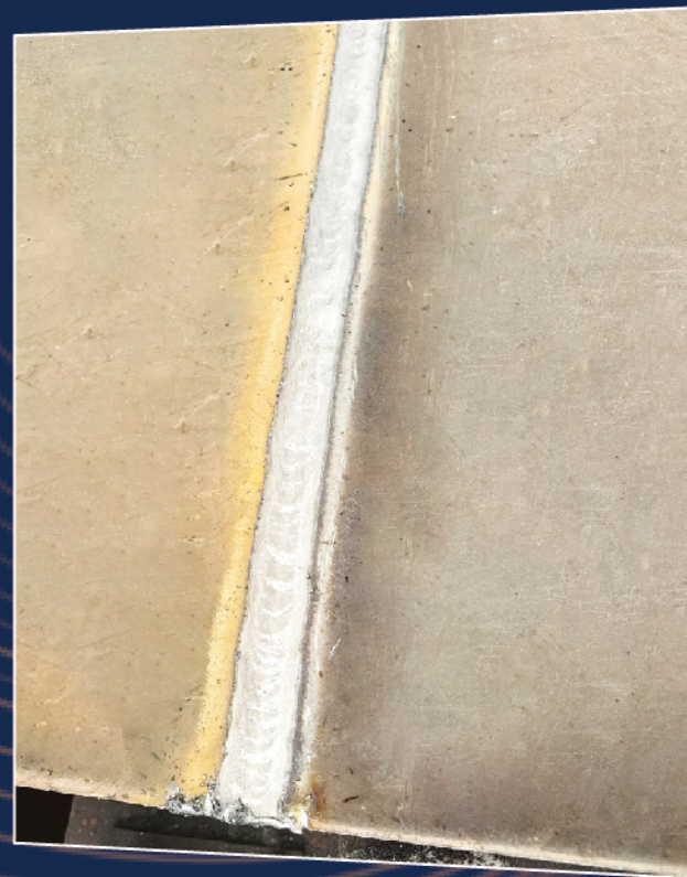
Main Girder Welding Process
